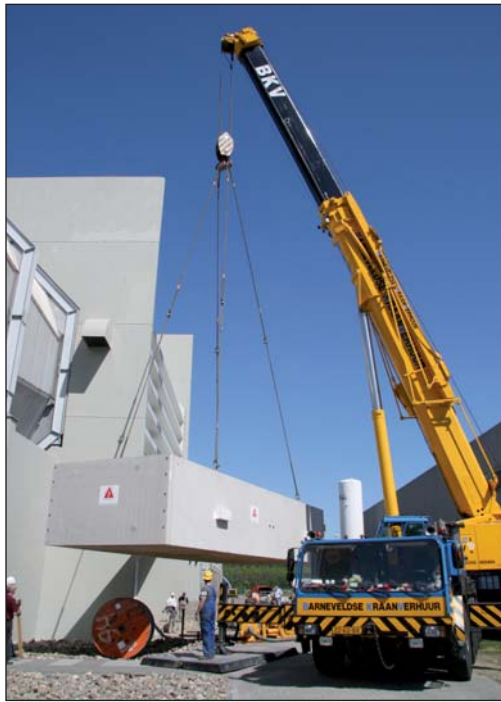
Figure 4: The cellar is lowered to its foundation next to the LLF
