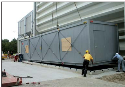
Figure 5: Placement of the fan controls container over the cellar
