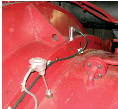
Figure 5: Vibration sensor (silver with dark cable) and temperature sensor (in front, grey cable) on the TWG compressor
